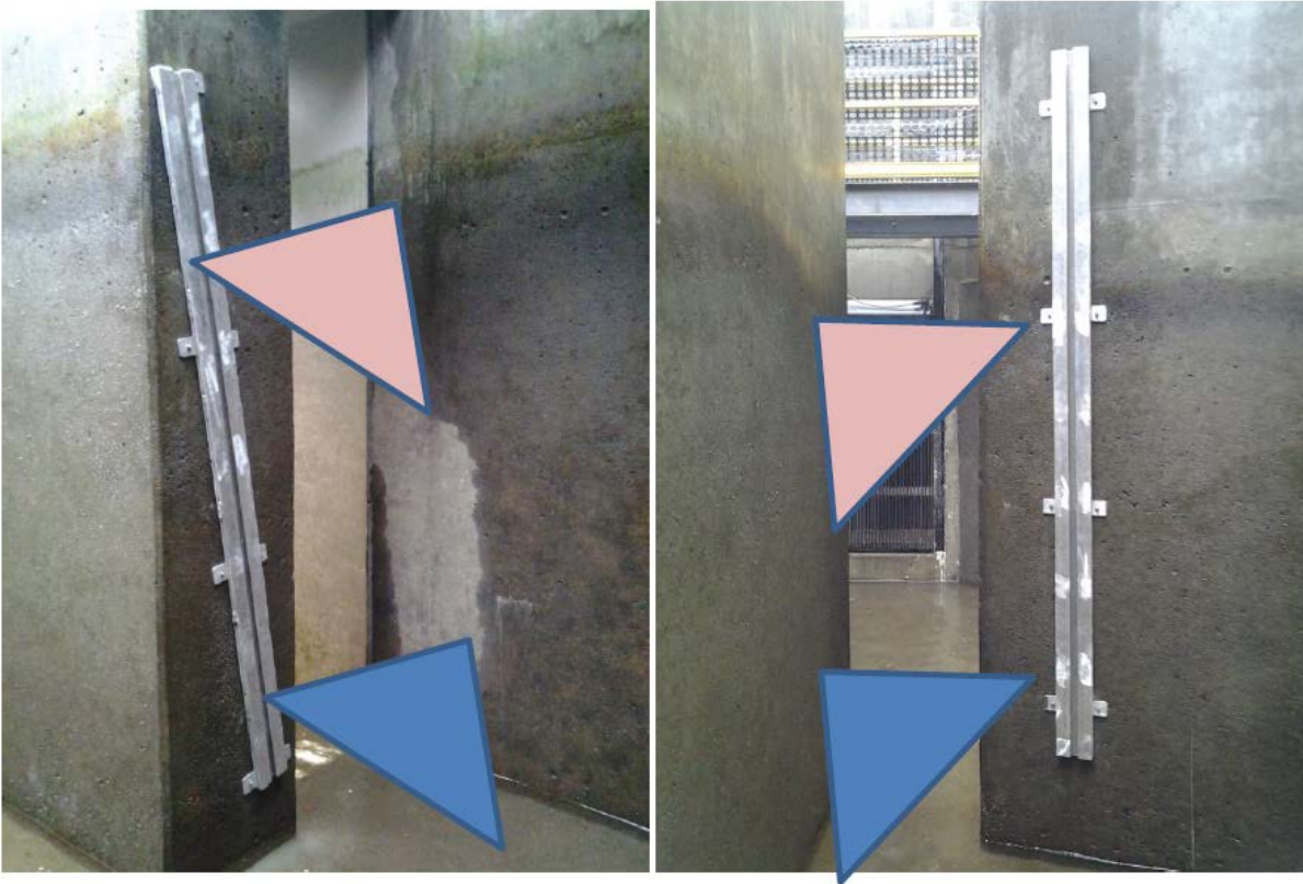
Figure 2. Examples of channels installed in Bradford Island Fish Ladder, February 2014. Blue triangles depict approximate fields of view captured by cameras in July 2014, pink depict proposed fields of view.
